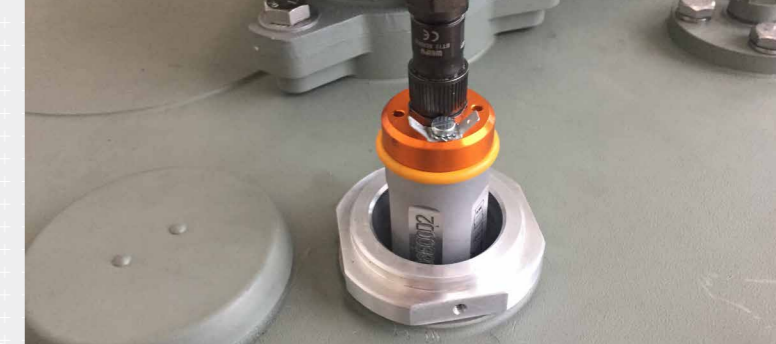
Figure 4. Installation in OLTP top hatch
